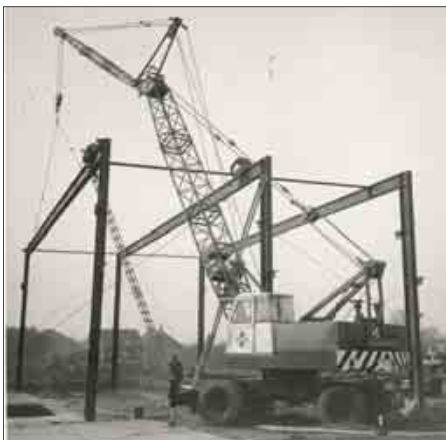
1972: rope-driven SK 15 with plastic operator cab
