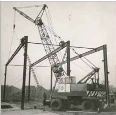
1972: Rope-driven SK 15 with plastic operator cab
